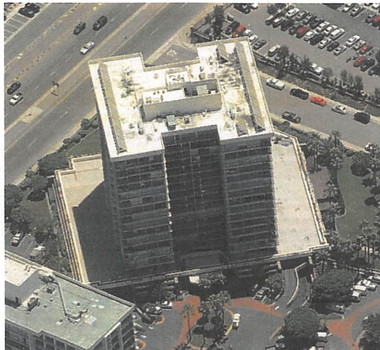
Figure 3-1 – Aerial View of the Site, Looking East (Microsoft Maps)
